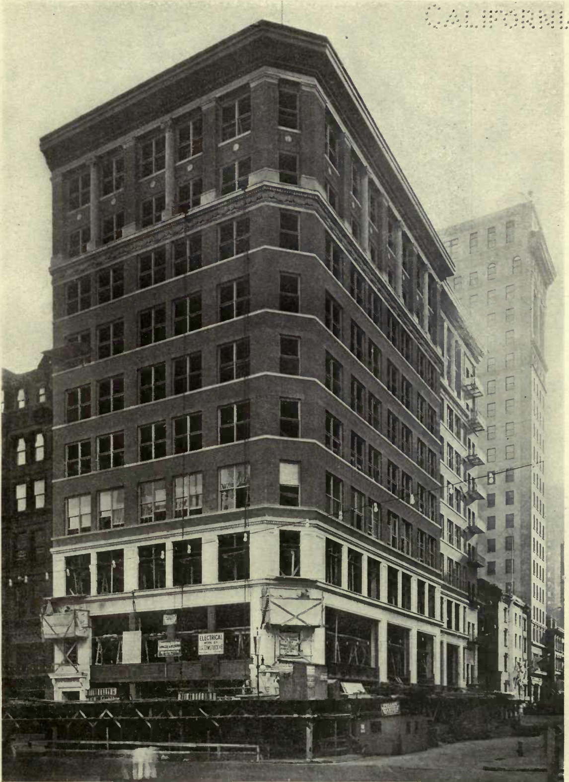
Rogers Peet Building, New York, N. Y. Townsend, Steinle & Haskell, Architects Basement waterproofed with Truscon Waterproofing Paste, Concentrated.
